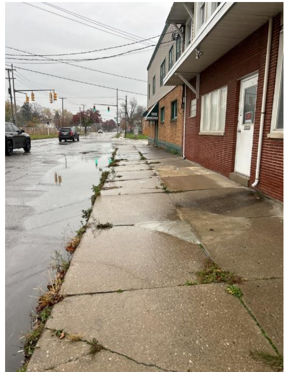
Figure 9 Clogged Road and uneven sidewalk
