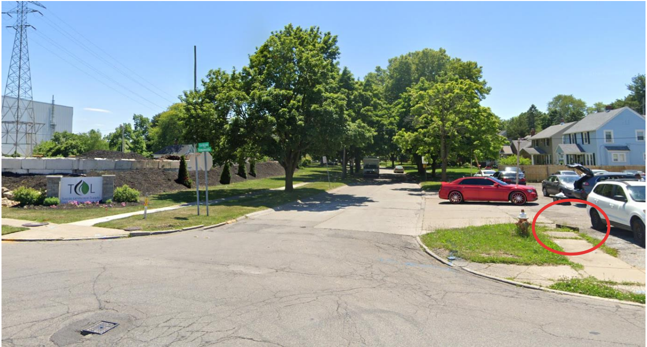
Figure 8 Missing ADA accessible ramps and raised manhole in middle of the sidewalk
